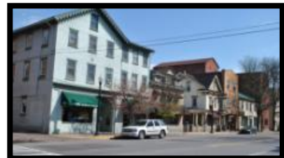
Mixed-use buildings create vibrant communities
