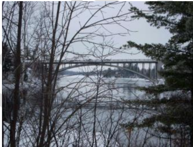
Figure 111: Keewatin Bridge (source: City of Kenora)
